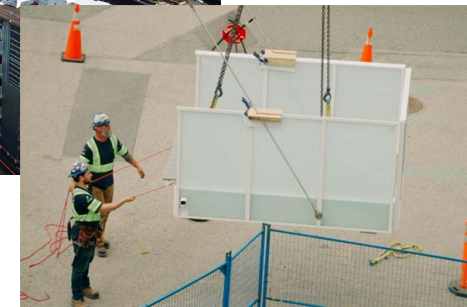
Clip On Balconies-Vienna House, Vancouver
