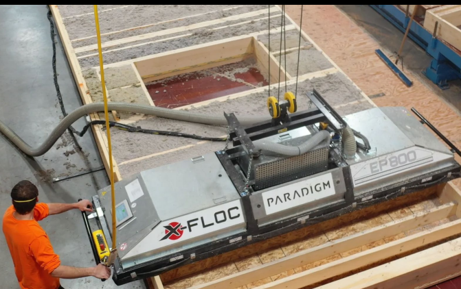
Paradigm Building Solutions - Louis Creek (Thompson Nicola)
