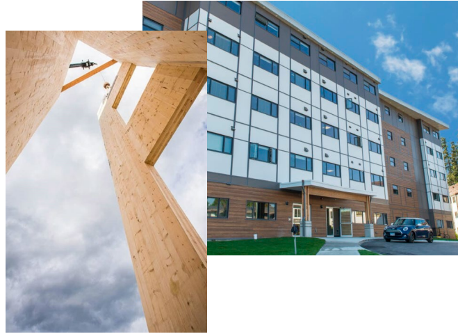
MT Elevator Shaft - Mercer, Okanagan Falls
