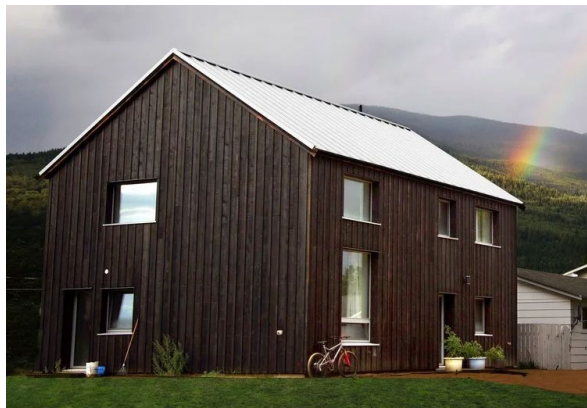
Valemount Passivhaus, 2016 (Roof & Wall Panels – Collective Carpentry, Invermere)
