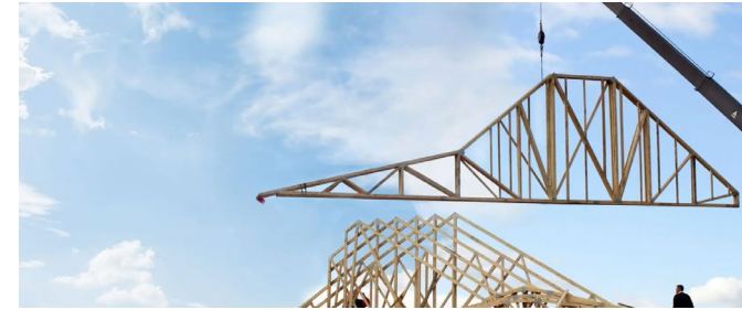
Prefabricated Roof Truss - Alliance, Abbotsford
