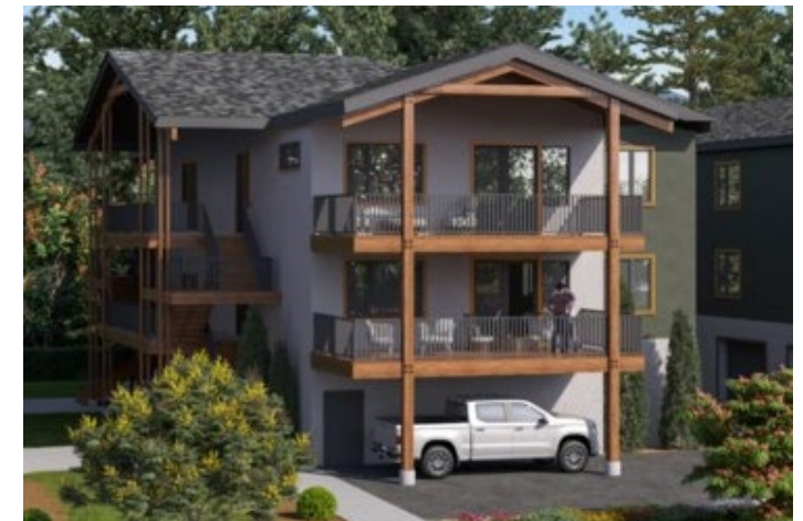
The Alders - Innovation Building Group, Pemberton, 2026 (Modules – Moduline, Penticton)
