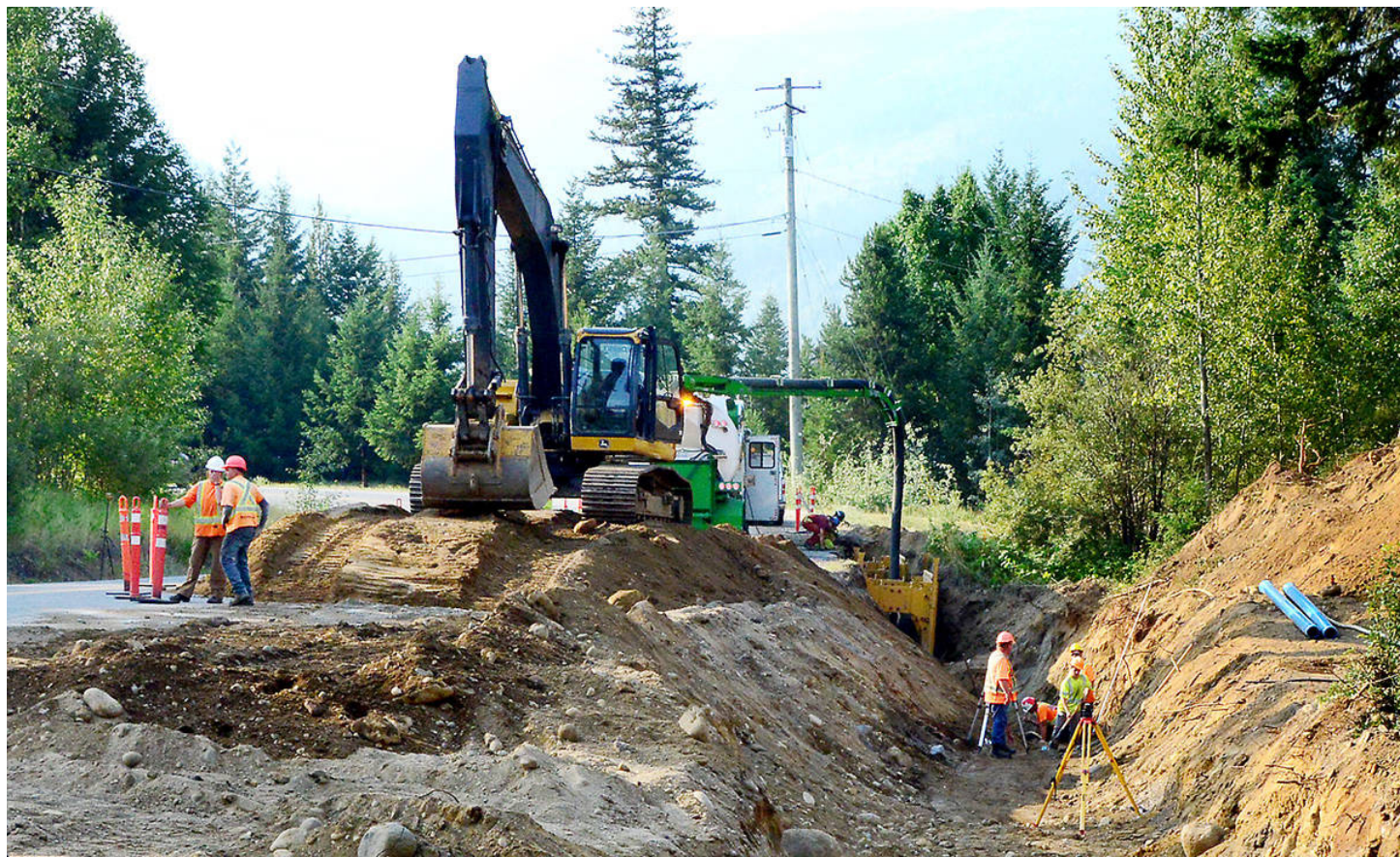
Drinking Water Excavation – City of Vancouver
