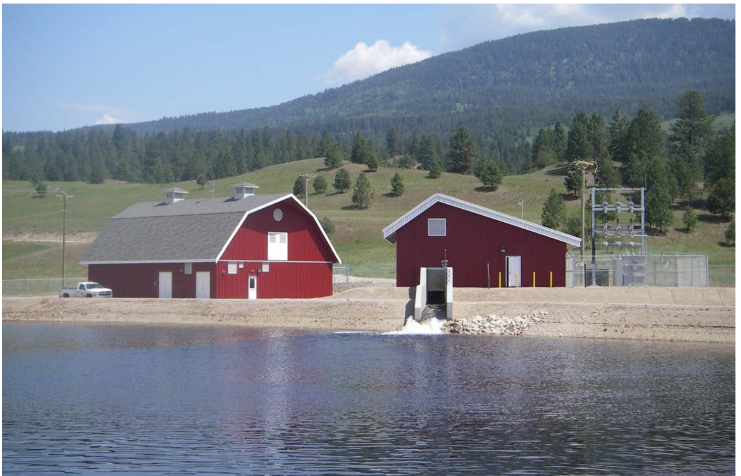
Hydroelectric generating station – District of Lake Country
