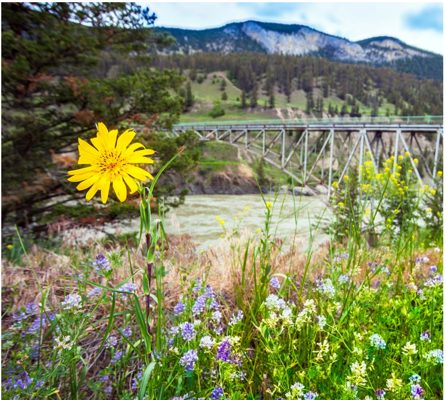
Bridge over the Fraser River - City of Williams Lake
