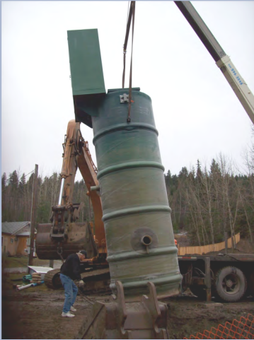
Installing a Sewer Lift Station at Pine Valley
